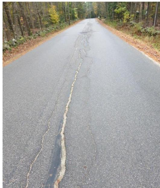
An example of Longitudinal Cracking
