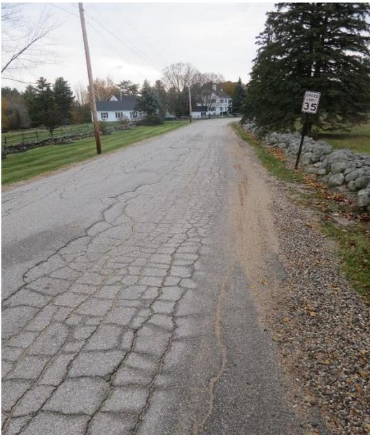
An example of Alligator Cracking
