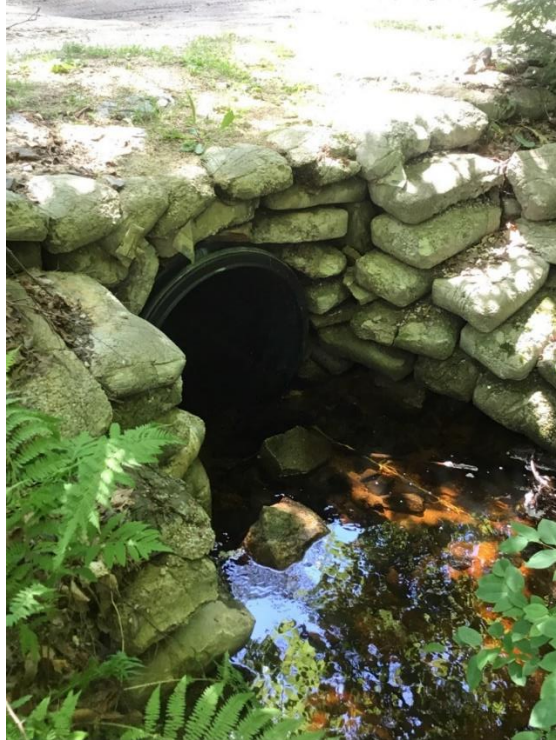
Figure C: Headwall (With Wingwalls) on Drake Ave Rd.
