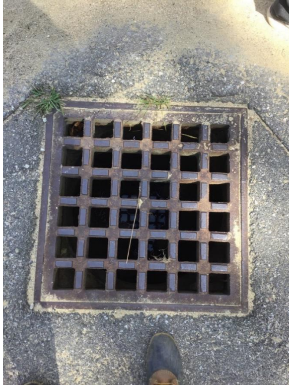
A. Catch Basin on Lakeshore Drive in Gilmanton, NH.
