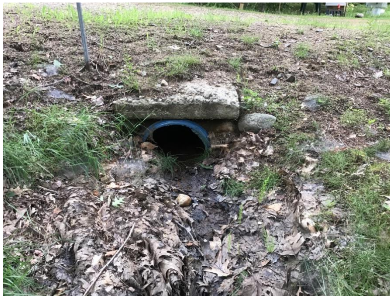
Figure B: Headwall (No Wingwalls) on Sawyer Lake Rd
