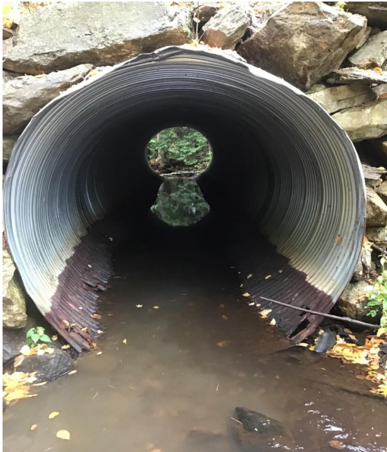
Loon Pond Road Metal Culvert in Gilmanton, NH.
