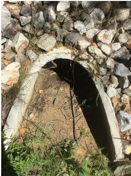
Figure A: Flared End Section on Stone Rd.
