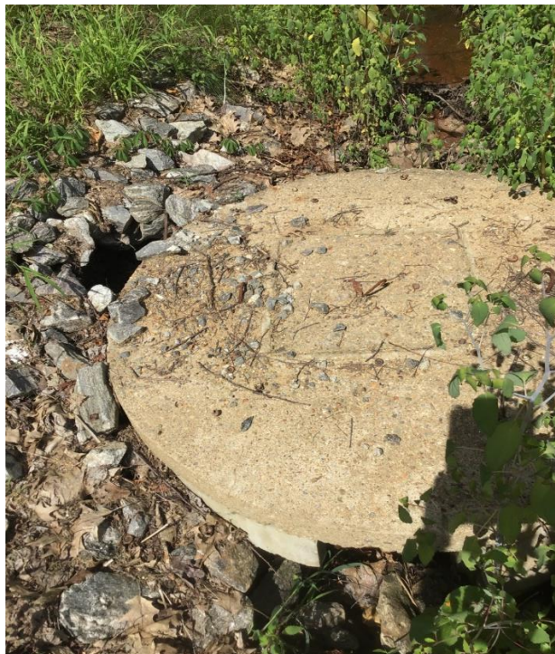
B. Drop Inlet on Currier Hill Road in Gilmanton, NH.
