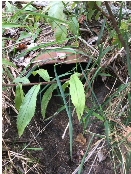
Figure D: No End Treatment on Allens Mill Rd
