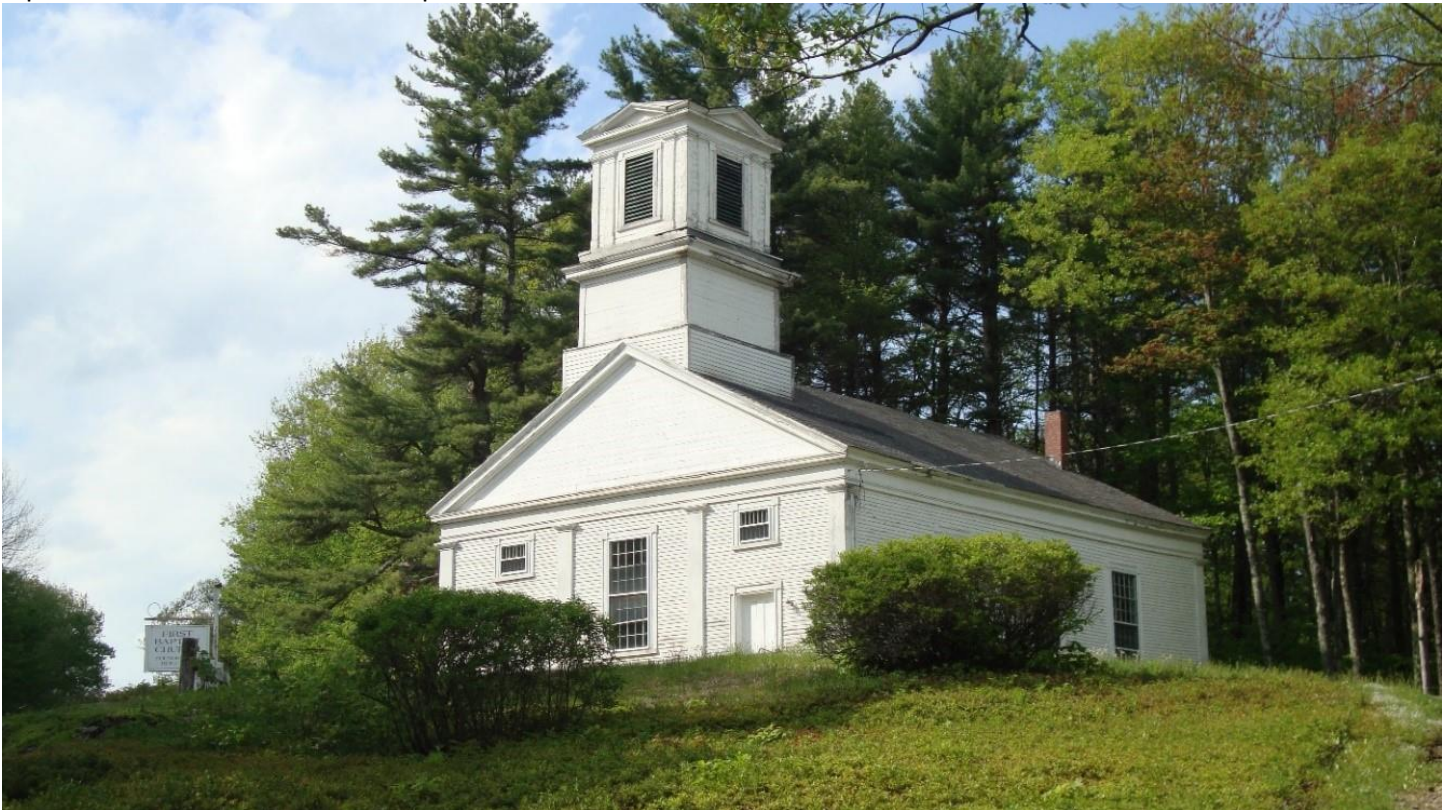
A portion of Condition Assessment photos
