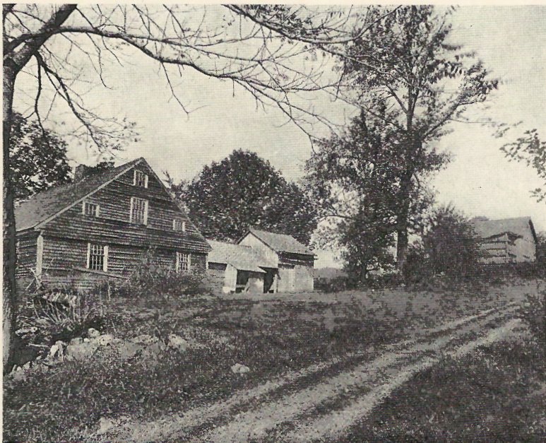
111. Abandoned farmstead in the Berkshires, typical of many back-country parts of New England
