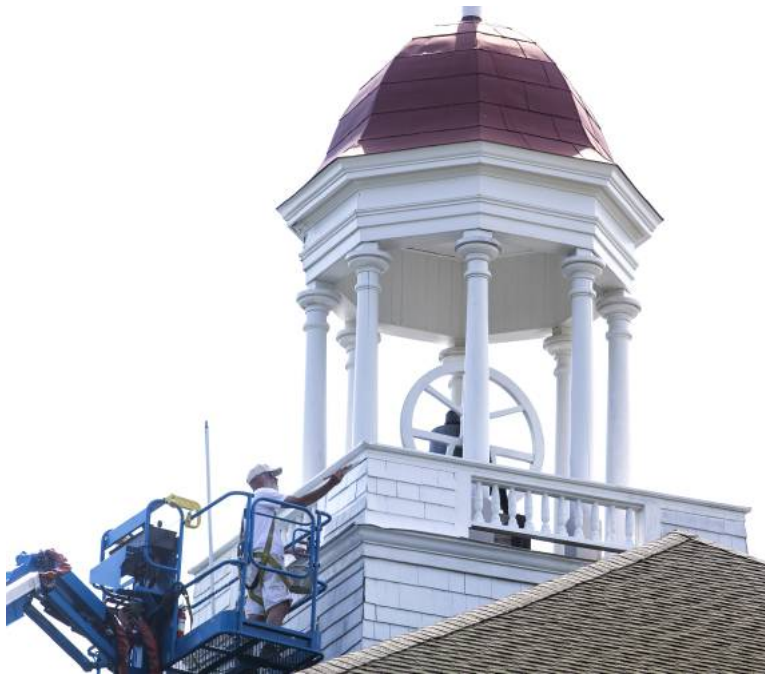
John Thompson of Laconia's J.L.T. Painting applies a coat of primer to the top of the Gilmanton office building.
