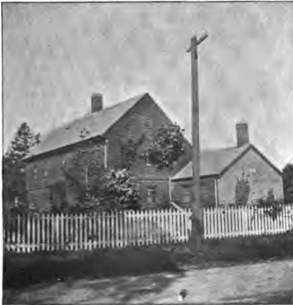
PILSBURY HOUSE RESTORED.
