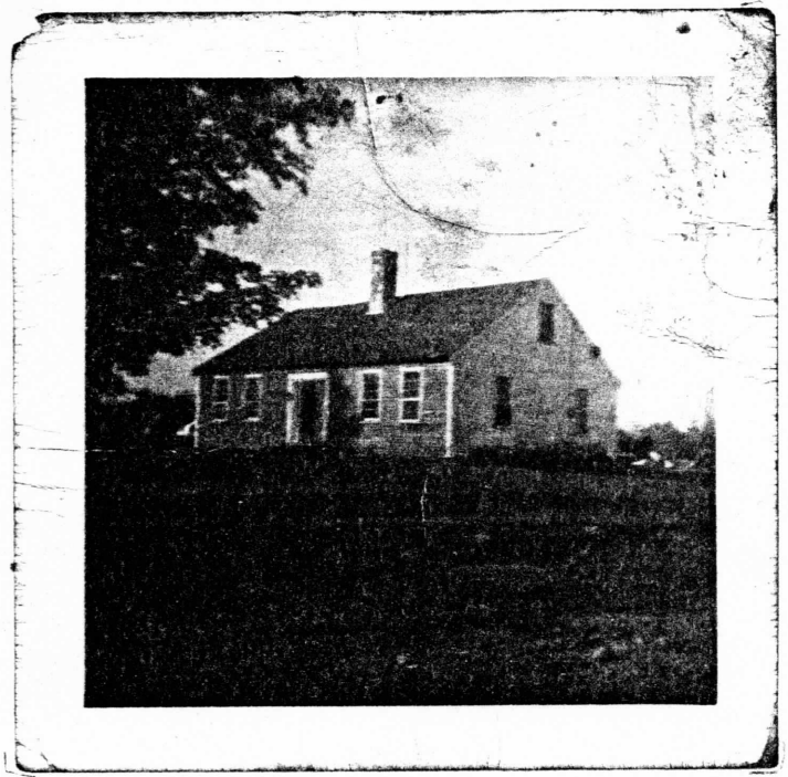
JONATHAN BUNKER-place ANDREW place , burnt in 1962
