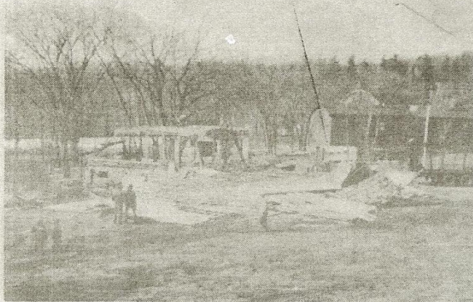
This is the same school about halfway through the demolition.
