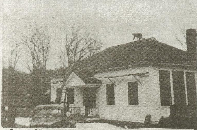
Former Gilman Iron Works School, turned over to the Fire Department, as the site for the new Fire Station to be built this year. This shows the beginning of the demolition.
