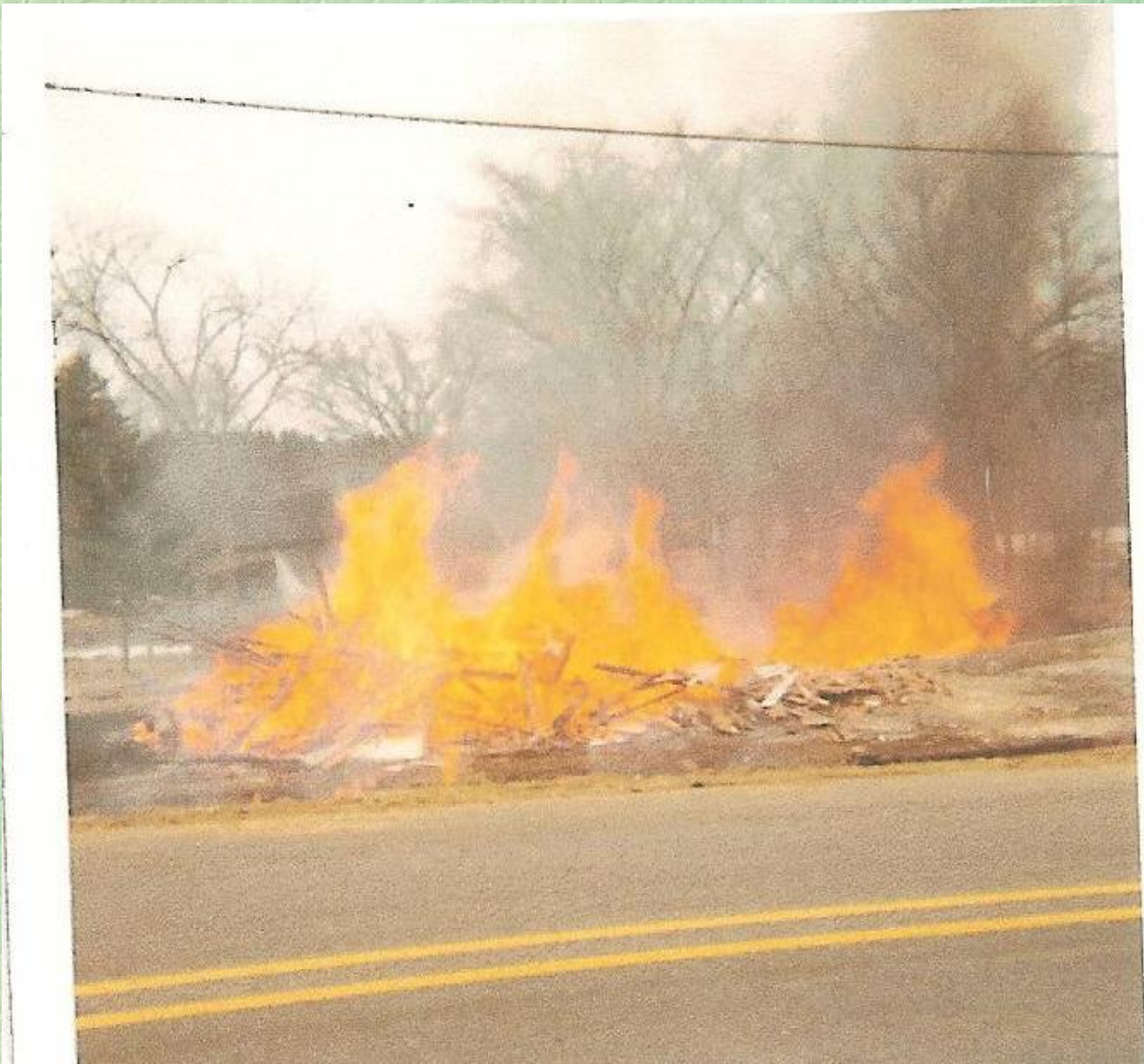
Schoolhouse demolition complete
