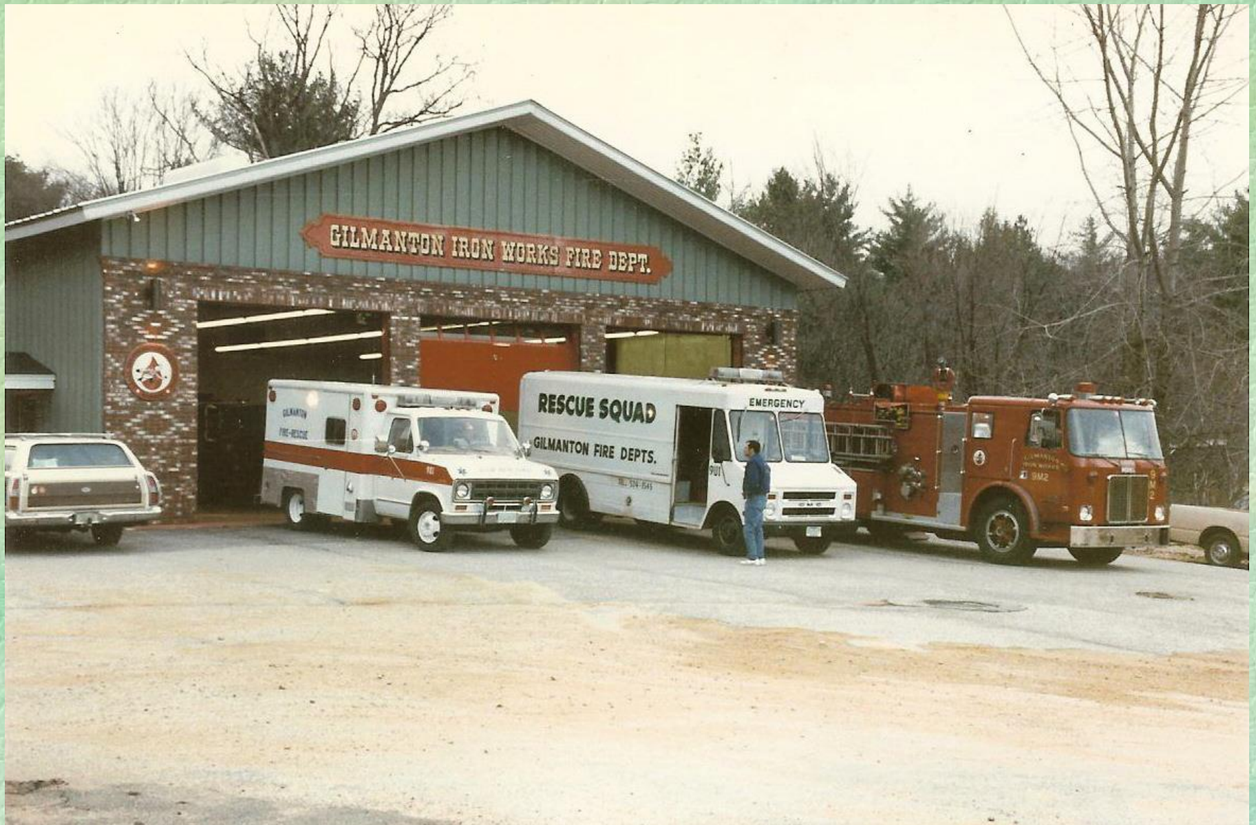
Completed IW Station
