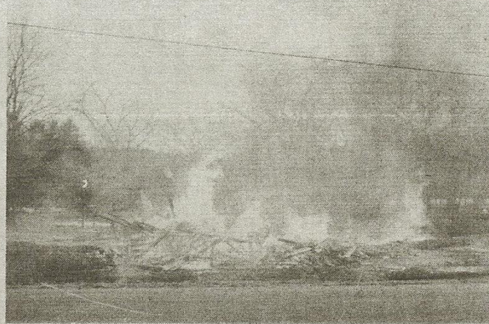
This is the end of the chapter for the old Iron Works Elementary School built over 50 years ago. Soon the New Iron Works Fire Station will be on this site.
