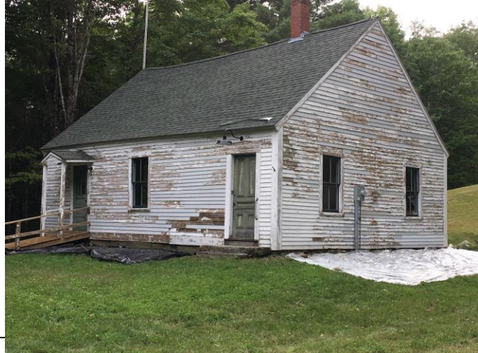
Removing Lead Paint
