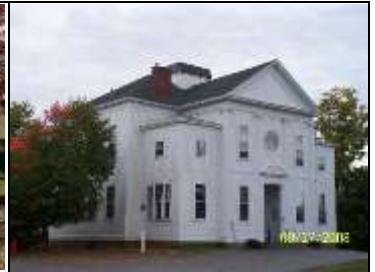
Cupola off for repairs 09/27/2008
